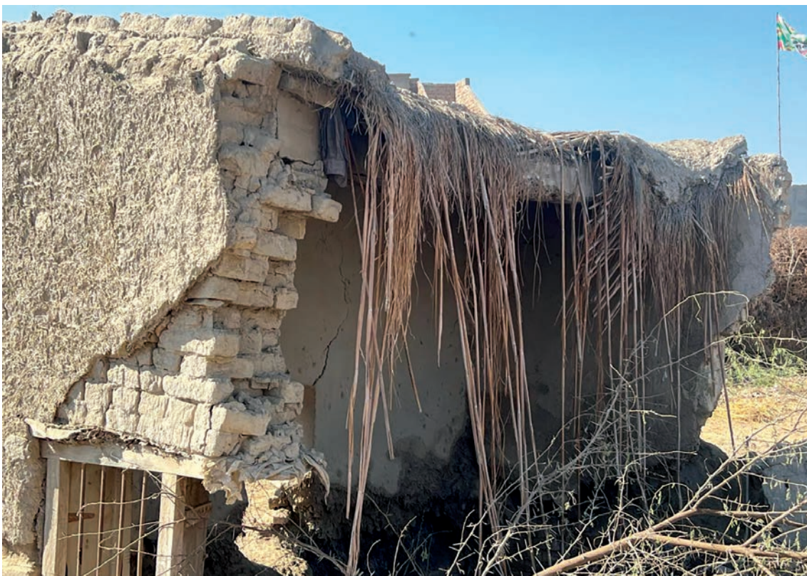
Flood-damaged traditional housing with collapsed roof demonstrates why many families were forced to accept inadequate SPHF housing despite its limitations
